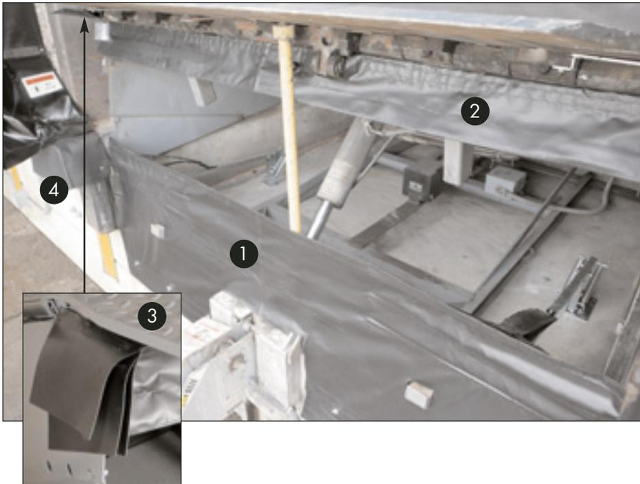
1. **The main sealing curtain** made of durable black vinyl is held in place by spring-loaded pivot arms and flexible stays that keep the seal engaged against the leveler and pit sides.
